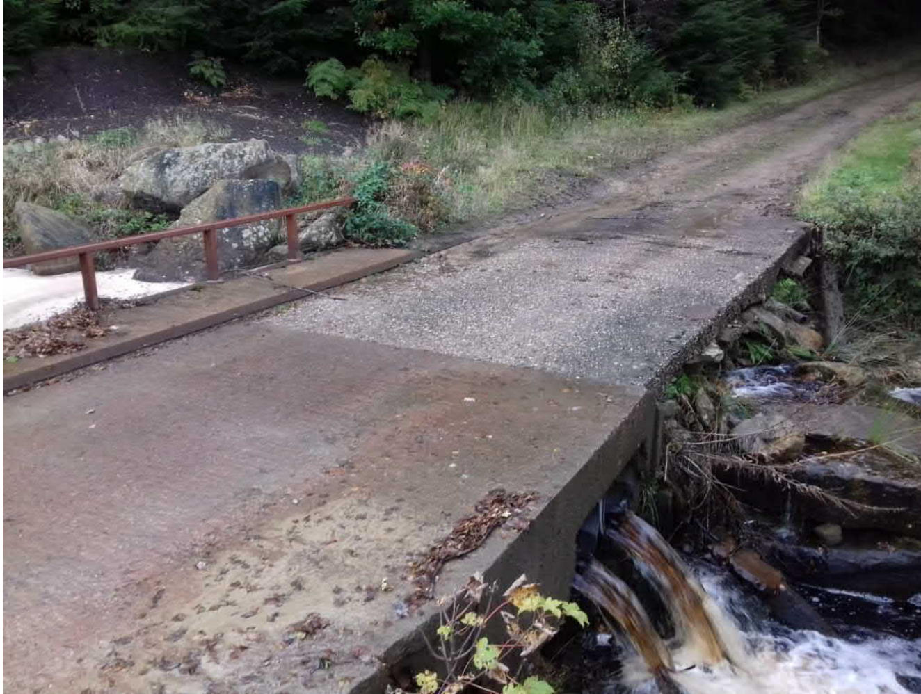
Photo 4 Low lying bridge
