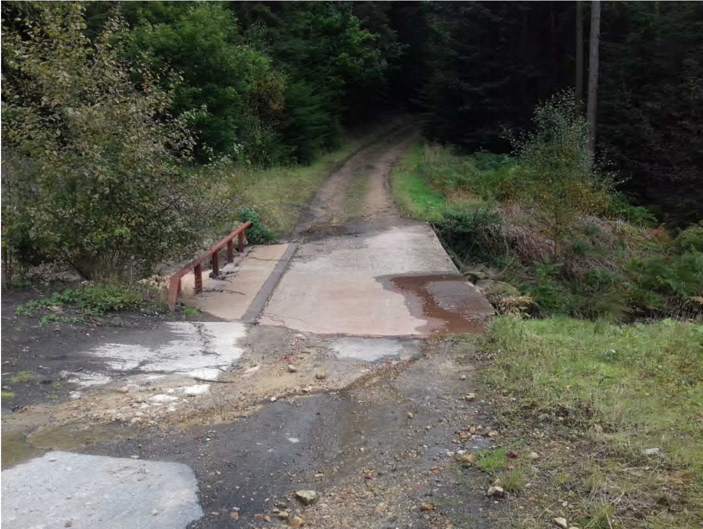
Photo 3 Low lying bridge
