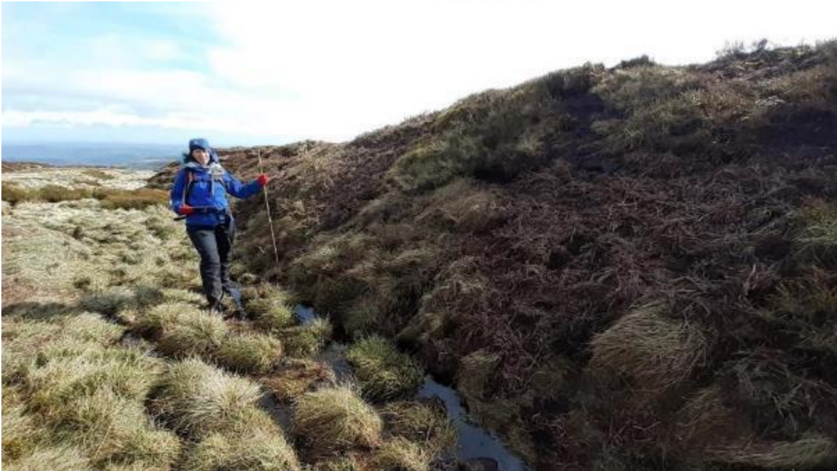
Photo 3 A 3m high slope reprofiled to greater than 45 degrees. There was sufficient existing vegetation to cover the reprofiled slope without the need for extensive bare peat restoration.
