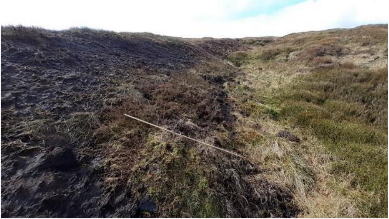
Photo 1 Photo showing translocated turf from the drip edge, now protecting the toe of the newly reprofiled slope. This gully is 2m high and has no evidence of water flow, therefore does not need extra toe protection.
