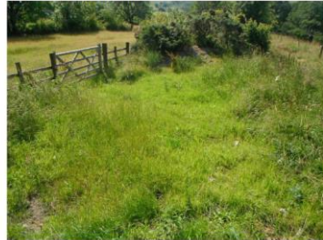
Photo 1: Downstream breach, Low Stanger Farm (source: West Cumbria Rivers Trust)
