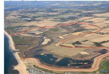
Photo 1: Medmerry managed coastal realignment site, 10 October 2013 (source: © Environment Agency and John Akerman ABPmer)
