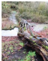
Photo1: Engineered dam 2 – attenuation and suspended sediment settlement during flood flows
