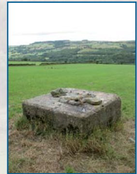
Concrete foundation for catenary defences. © photograph Christine Handley
