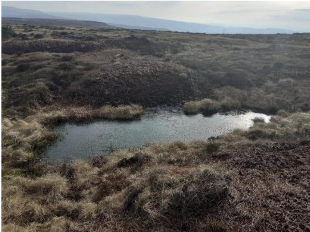
○ ○ Figure 20 Example of Gully block pool – peat dam on left. Dams can be stone, timber, plastic, heather bale or coir log.
