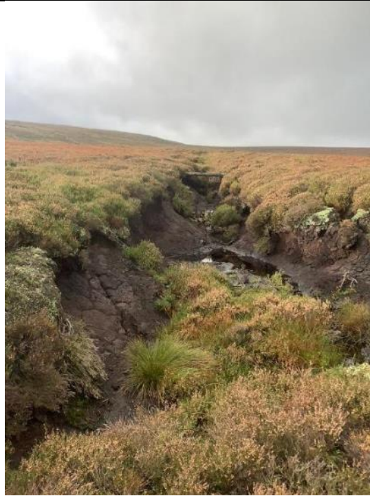
Photo 2 Photo showing steep eroding “grip” sides requiring re-profiling. Existing stone dams are visible within the grip in the background (looking upstream).
