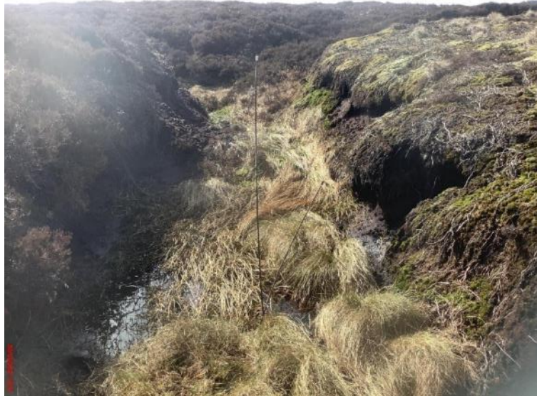
Photo 7 Photograph showing typical location for timber dam at Snailsden
