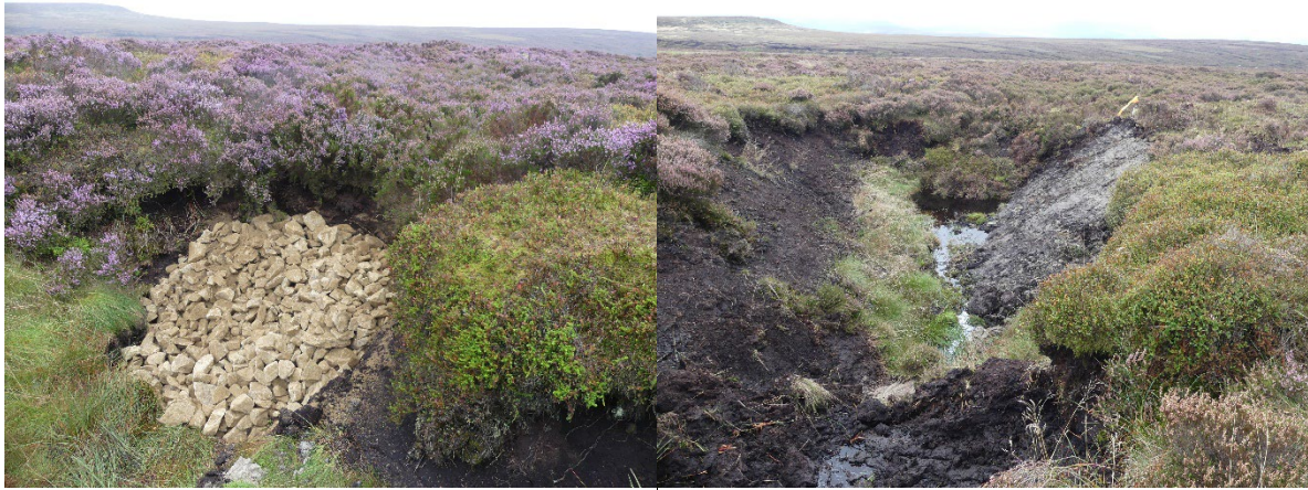
Fig. 10. Photographs showing the blocking process using a stone core at P2.1
