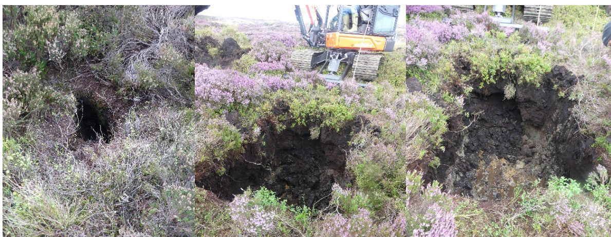
Fig. 9. Photographs showing preparation for blocking within a vertical “vent” hole
