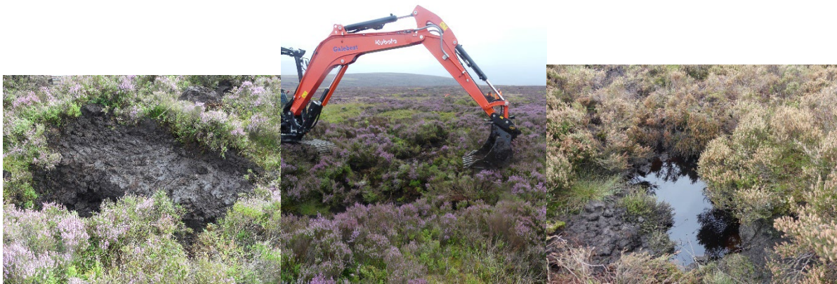
Fig. 11. Photographs showing the blocking process using a peat core at P1.4
