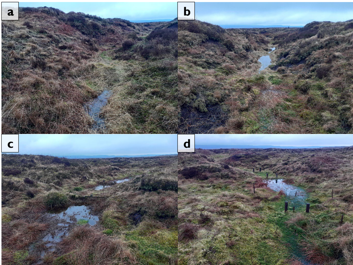
Figure 11: Gully blocks at mini-catchment N in varying states of maturation (February 2022) a) stone blocks partially sedimented, creating semi-permeable dam with temporary water storage capacity; b) stone blocks fully sedimented, creating minimally-permeable dam with long-term pool and minimal available temporary storage capacity; c) timber dams with gaps between planks partially sedimented, creating semi-permeable dam with temporary water storage capacity; d) timber dams with gaps between planks fully sedimented, creating minimally-permeable dam with long-term pool (full of Sphagnum) and minimal available temporary storage capacity
