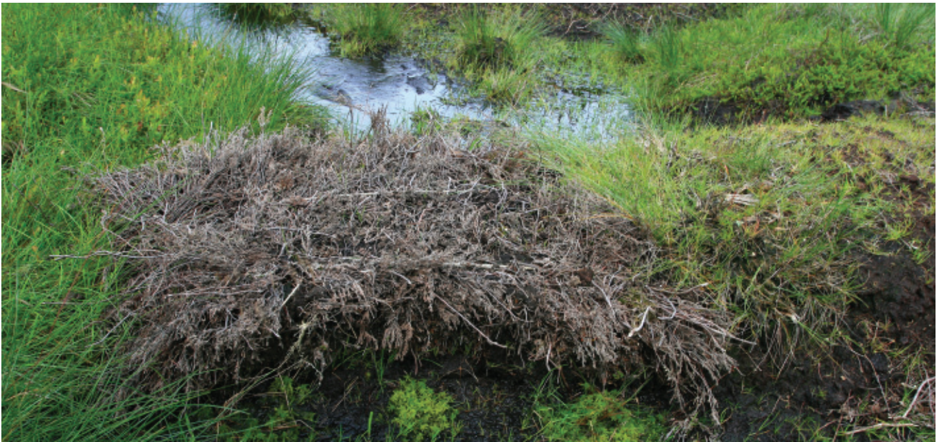
Figure 2: Shallow gully system, shortly after heather bale dam installation
