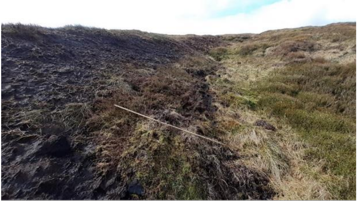
Photo 1 Photo showing translocated turf from the drip edge, now protecting the toe of the newly reprofiled slope. This gully is 2m high and has no evidence of water flow, therefore does not need extra toe protection.
