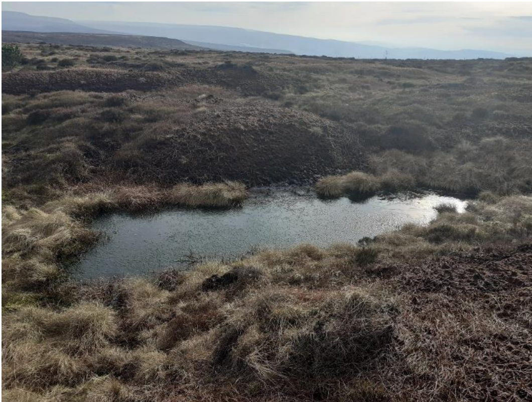
Figure 30:6 Example of Gully block pool - peat dam on left. Dams can be stone, timber, plastic, heather bale or coir log.
