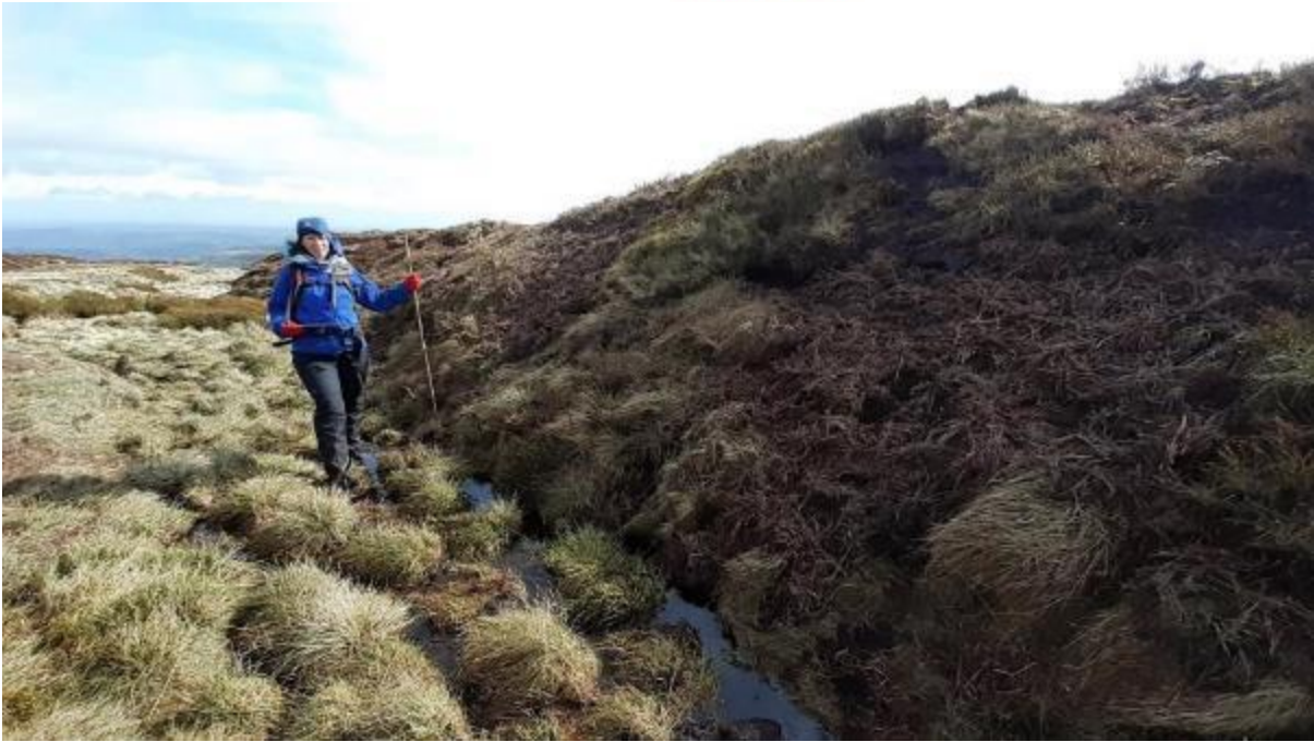
Photo 3 A 3m high slope reprofiled to greater than 45 degrees. There was sufficient existing vegetation to cover the reprofiled slope without the need for extensive bare peat restoration.
