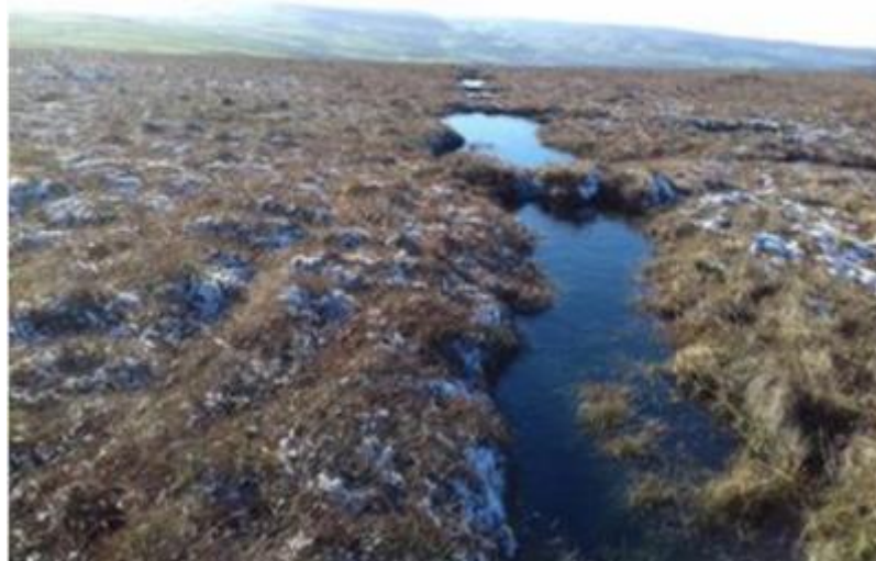
Figure 15 A borrow pit in the top right 3 months post construction
