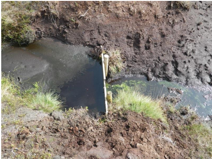
Figure 8.14: Overlap fencing dam (number 83) at Upper North Grain in September 2014
