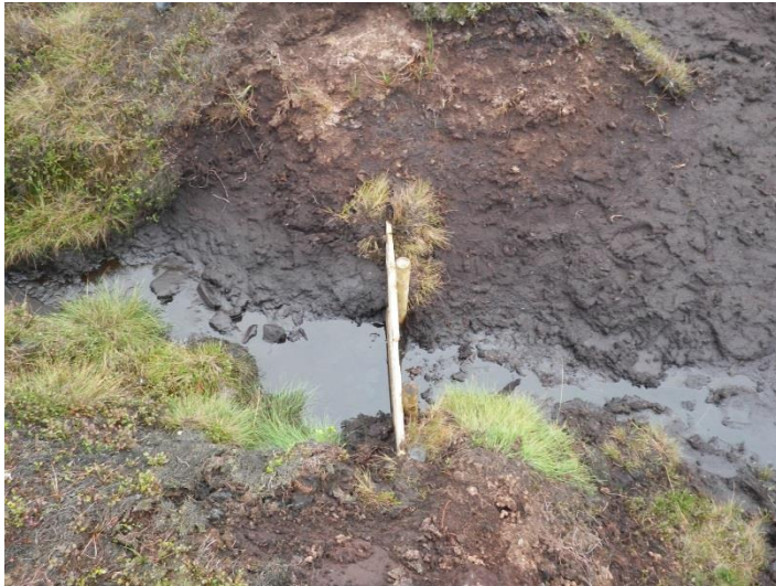
Figure 8.13: Overlap fencing dam (number 83) at Upper North Grain in September 2013
