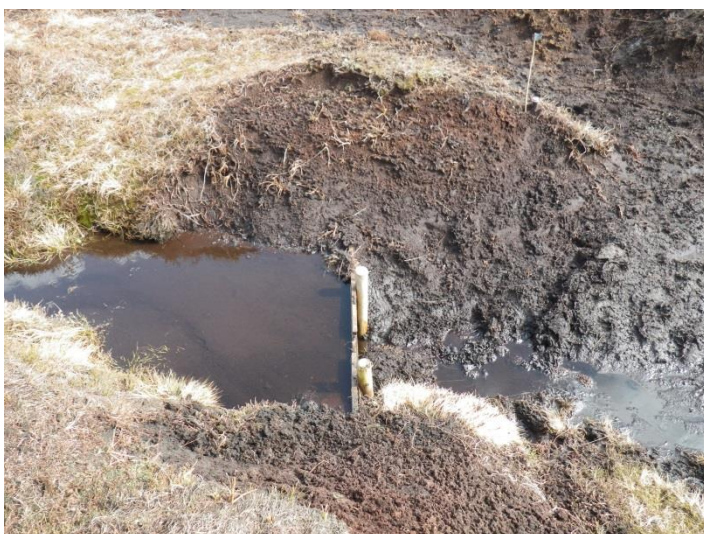
Figure 8.15: Overlap fencing dam (number 83) at Upper North Grain in March 2015
