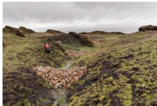
Early stage restoration
