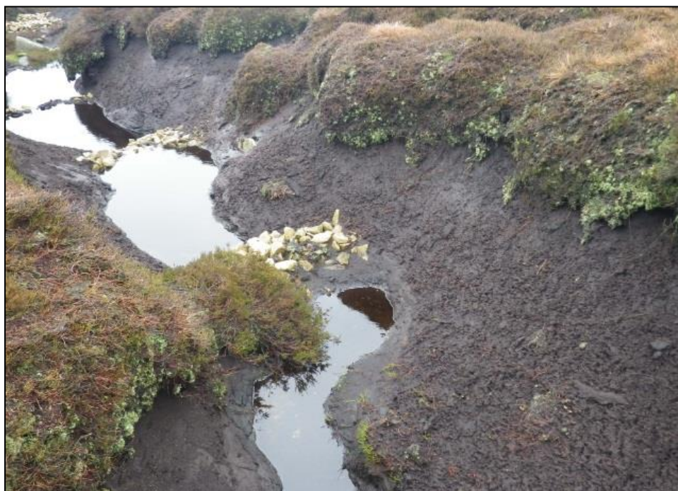
Figure 11 – Photograph of a gully block at System 2 taken at time of surveys two weeks after gully block installation in November 2012 (a); and fifteen months after gully blocking in February 2014 (b).
