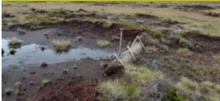
Slowing water movement across bare peat surfaces using heather bales or coir rolls. This helps stabilise the peat by reducing the erosive forces of the water and by capturing particulate peat allowing species like cotton grass to act as initial colonisers. Sphagnum can be added following stabilisation
