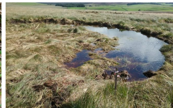
Bunds – Semi-circular raised mounds are created out of peat, in order to trap water and raise the water table.
