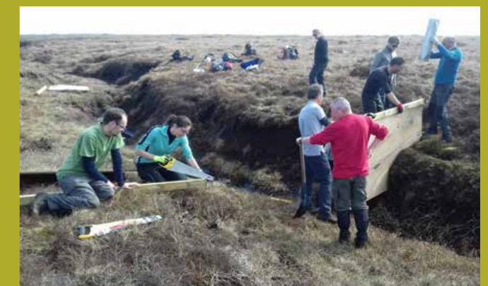
Staff and volunteers installing v-notch weir
